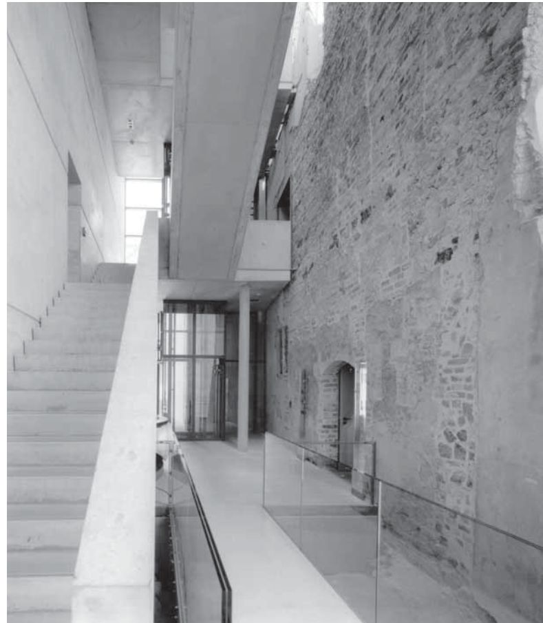
Entrance hall of the Lutherhaus in Wittenberg: View of the west pediment and the foundation of the Lutherturm.
